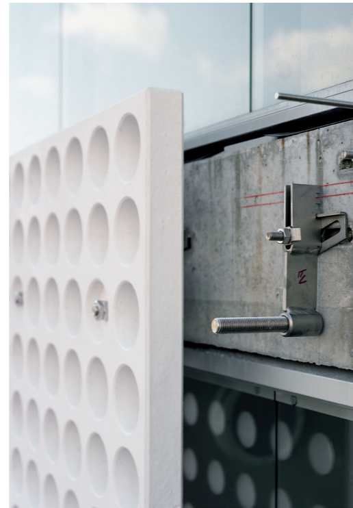
550 m 2 fibreC 3D elements with a thickness of 7 cm are cladding the Lontoonkatu 9 project in Helsinki, designed by Kirsi Korhonen and Mika Penttinen Architects. The entire facade was divided into 16 different types of panels with lengths up to 3.8 m. More than 400 concrete elements with faced concrete quality on both sides offer an interesting view from inside of the building.
