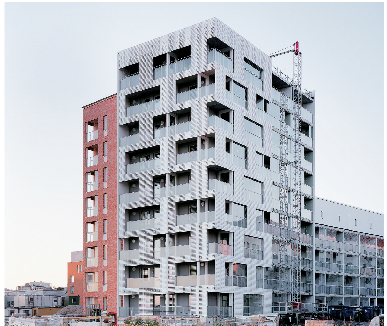
550 m 2 fibreC 3D elements with a thickness of 7 cm are cladding the Lontoonkatu 9 project in Helsinki, designed by Kirsi Korhonen and Mika Penttinen Architects. The entire facade was divided into 16 different types of panels with lengths up to 3.8 m. More than 400 concrete elements with faced concrete quality on both sides offer an interesting view from inside of the building.
