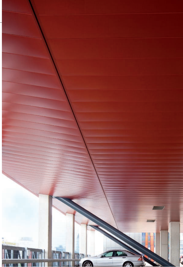
Above : Red Apple, Rotterdam, The Netherlands Product : Wide Panel 300C/300L Exterior Ceiling Architect: KCAP Architecten & Planners
