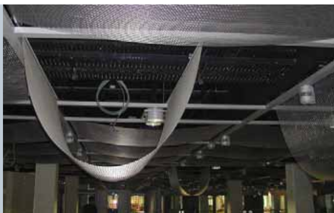
Mesh inserted into a slot profile
