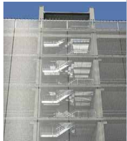
Project: Car Park 3–Airport Nuremberg, Nuremberg, Germany, Architect: Kappler Architekten
