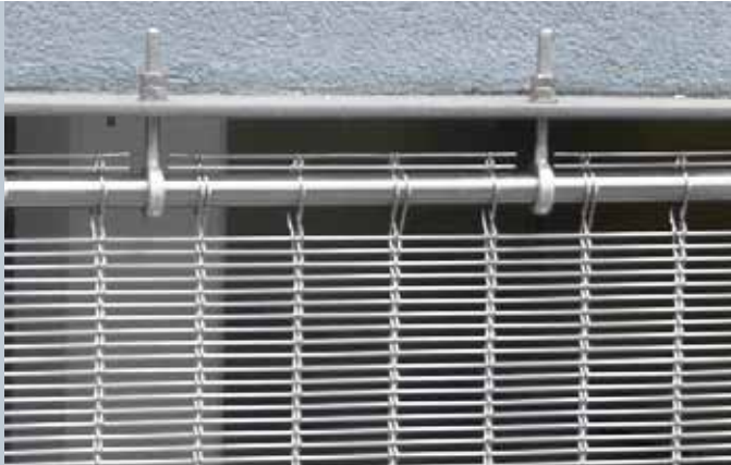
Top mounting: round rod with eyebolts
