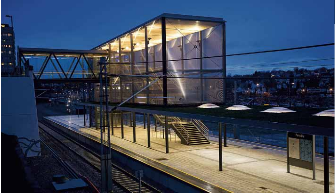
Project: Paradis Stasjon, Stavanger, Norway, Architect: Birger Heyerdahl
