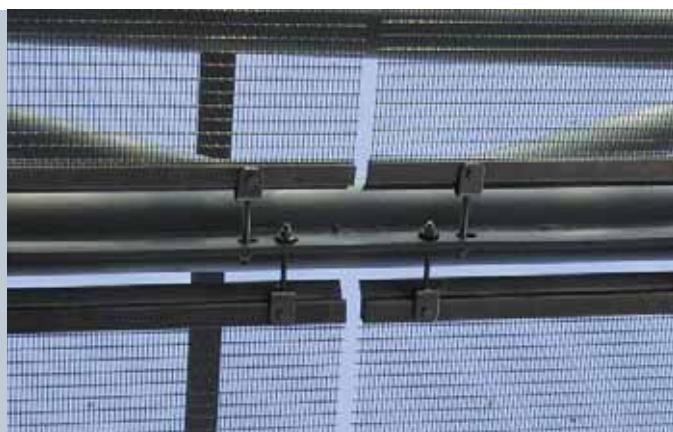
Mesh with flat tension profiles and clevis screws
