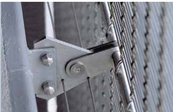
Intermediate mounting: round rod with pendular clips
