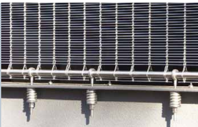
Bottom mounting: round rod with eyebolts and pressure spring
