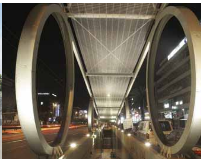
Project: Siggrou Avenue, Athens, Greece Architects: YPEHWDE planning unit
