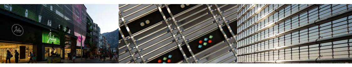
IMAGIC WEAVE® transparent media façade, a combination of HAVER Architectural Mesh and the latest LED technology of Traxon Technologies, creates with an infinite number of colours individually programmable lighting effects including full video content on new or existing façades.
